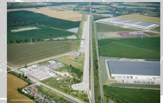
Triple Crown Intermodal Facility
